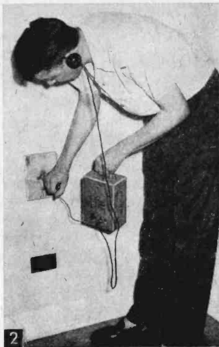
Fig. 1. Utility shut-off valves, tanks and shallow cables buried under asphalt, concrete or soil are located by whistle in headphones. Fig. 2. Using locator to trace route of electrical wiring or plumbing concealed in walls or floors, prior to making home repairs or alterations requiring cutting into walls.
